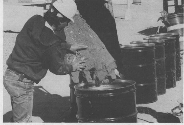
BOLTS AND DIRT exhumed from a construction trench inside Tech Area 1 are guided into 55-gal. drums by a member of a contract construction crew. Because some of the counterfeit bolts were plated with cadmium, the bolts were sifted from the dirt and sent to a hazardous waste disposal facility in Louisiana.
